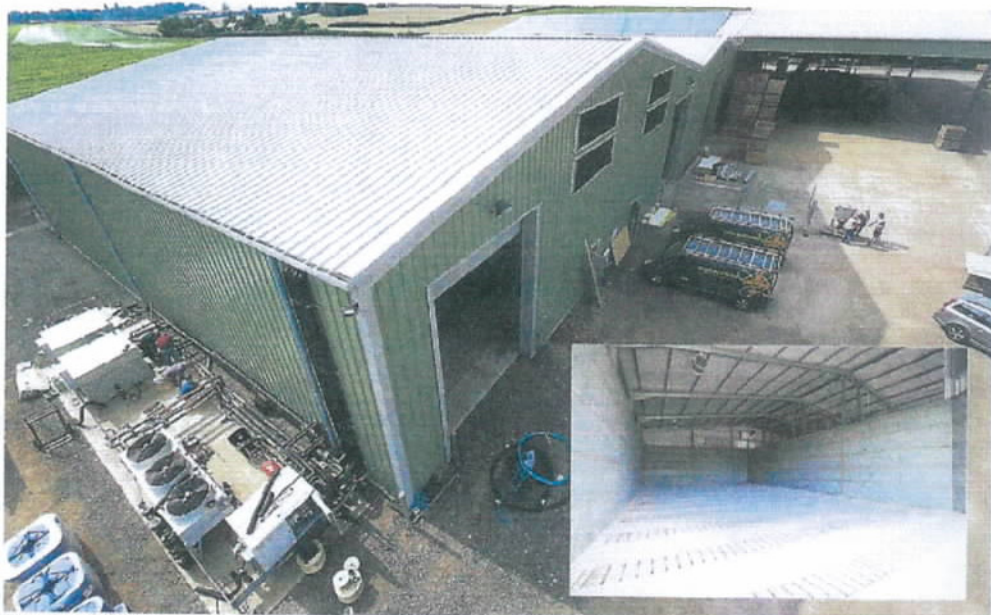
The new 2,600-tonne store is capable of working at high temperature and low humidity or vice-versa.
